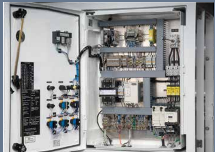
Interior door / electrical
